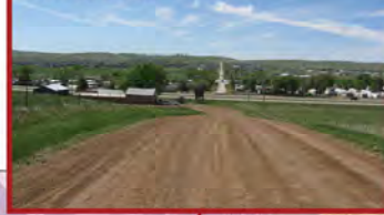
Significant Grade Differential
